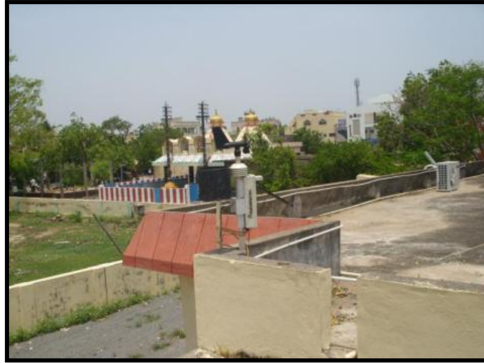
Figure 5-1: Automatic weather station installed at Thullur
